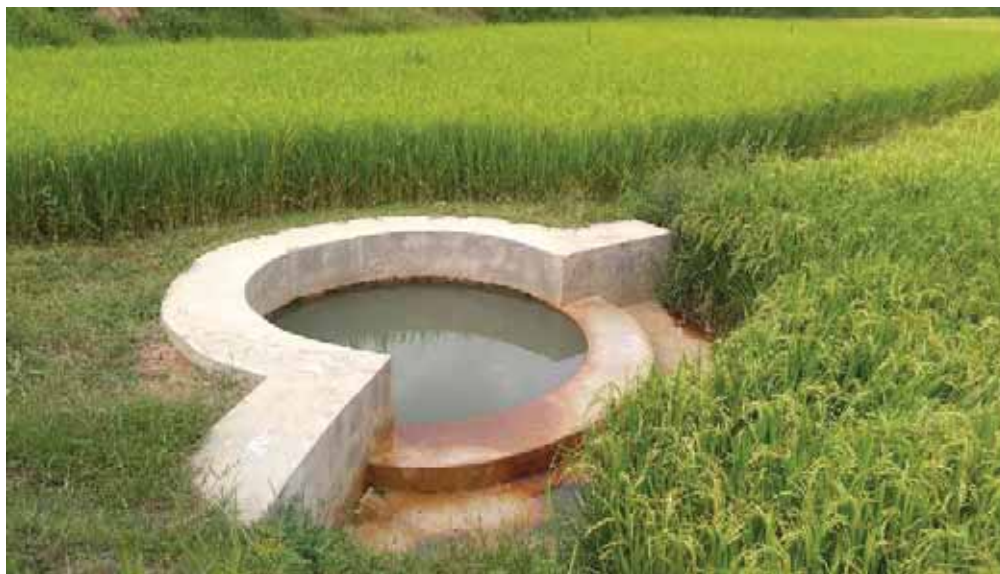
Shallow Well Constructed at Sisai, Gumla
