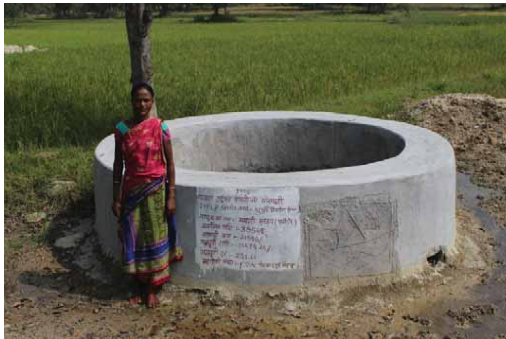
Shallow Well Constructed at Potka, East Singbhum
