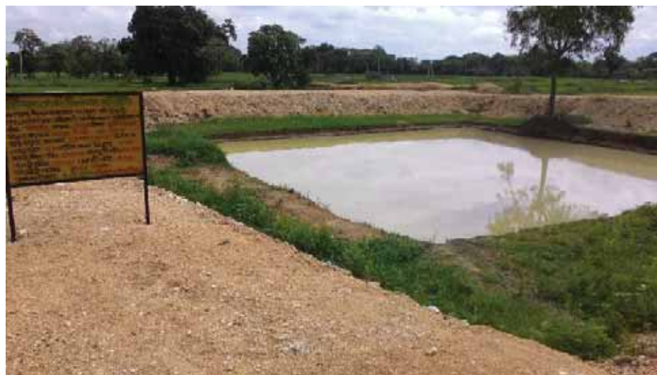
Pond constructed at Potka, East Singbhum
