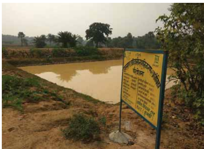
Pond constructed at Sundarpahari, Godda
