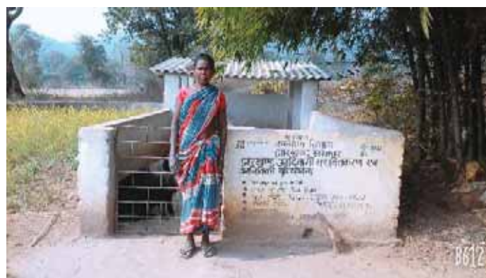
Low cost Pig Shed
