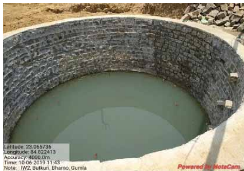
Irrigation Well Constructed at Bharno, Gumla
