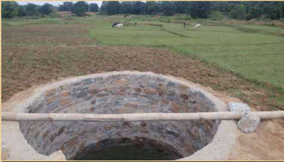
Shallow Well Constructed at Toto, Bhandra, Lohardaga
