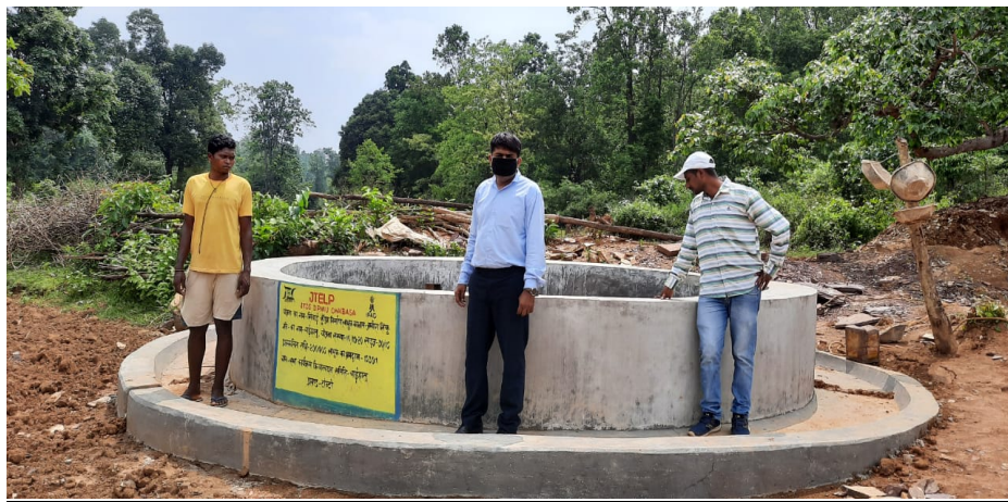
Irrigation Well Constructed at Baihatu, Tonto, West Singhum
