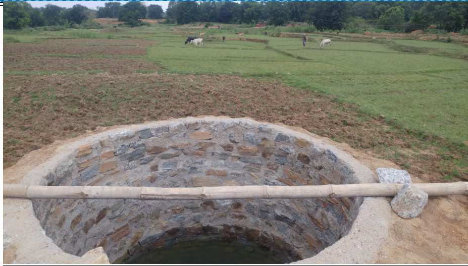
Shallow Well Constructed at Toto, Bhandra, Lohardaga
