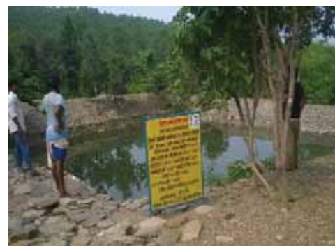
Constructed pond at Potka
